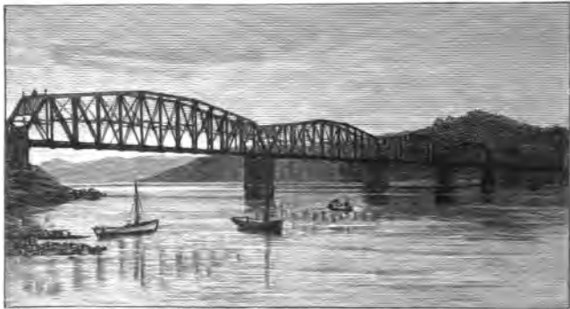
FIG. 31.—BRIDGE OVER THE HAWKESBURY RIVER, 3000 FEET LONG.
